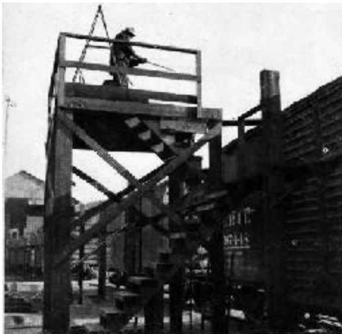
Joseph Caputo, carman at Dumore car shops, suggested building this platform along the ear repair track to facilitate riveting and repairing box car roofs. Rivet forge is set up on platform, which is slightly higher than car, and rivets thrown to riveter working on any part of roof
