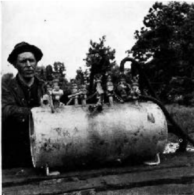
William Buchheister, steel foreman in the Department of Structures, welded several nipples with valves and standard air line fittings to pressure tank from which as many air tools can be operated at same time. Only one long hose needed from compressor to tank. Saves air hose, tools work better
