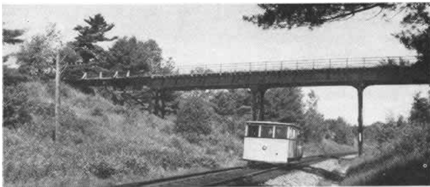
RUBBER BRIDGE is so called because it has had to be stretched as the embankments changed shape. Note the new approaches.
