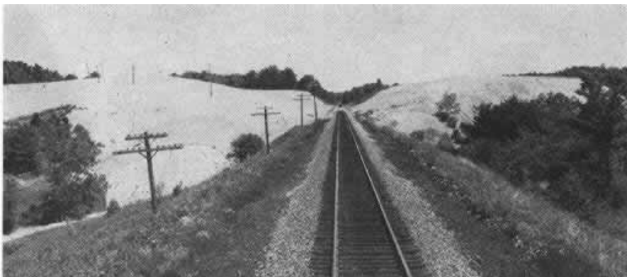
HERE AT HOTCHKISS CUT the banks have been all but leveled to prevent their movement toward the River Line track.
