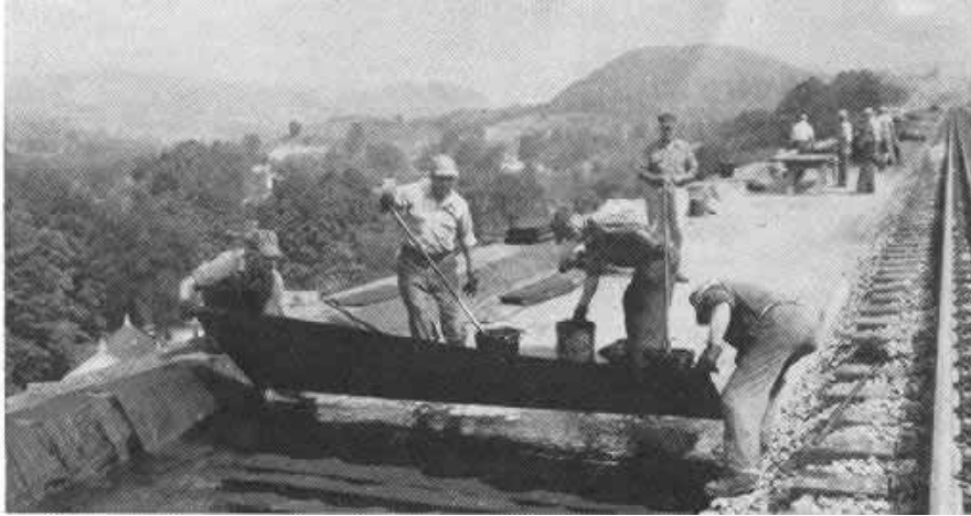
FABRIC SATURATED WITH asphalt was laid on the bridge deck.
