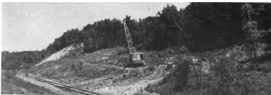
A DRAGLINE KEEPS THE CLAY BANKS of Tunnel Cut No. 2 from sliding across the tracks and closing the River Line,
