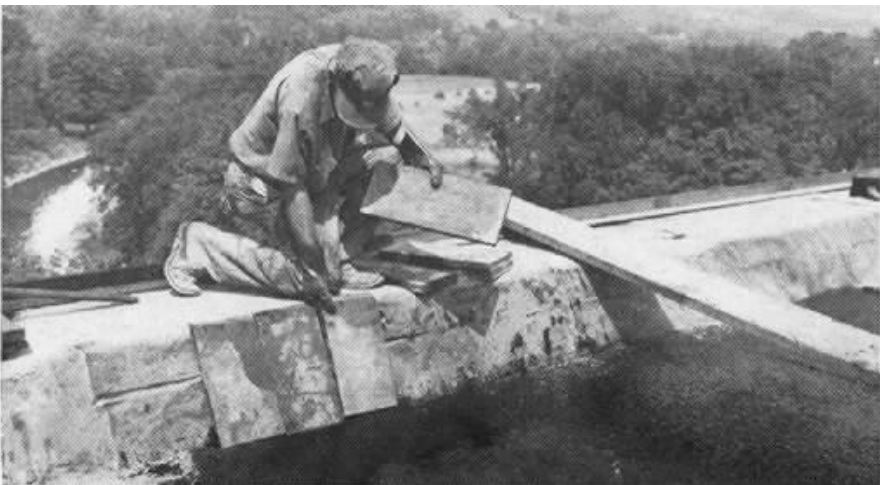
ASPHALT PLANK was placed on the inner faces of the parapets.
