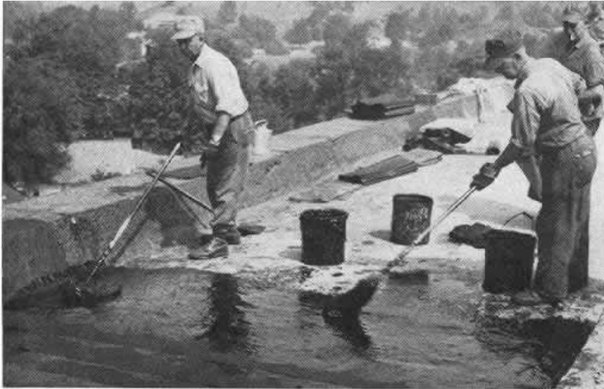
A LAYER OF HOT ASPHALT was mopped over the fabric.
