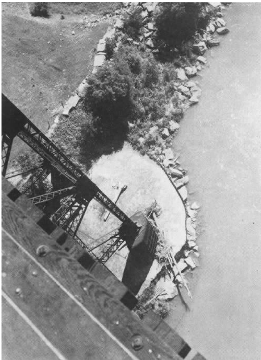
A DIZZYING DISTANCE BELOW THE RAIL, thousands of tons of rip-rap and concrete make a solid pier for Belfast Viaduct.
