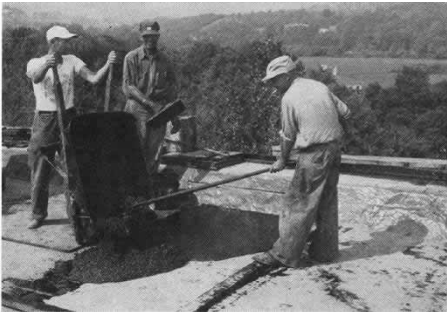
HOT MASTIC WAS POURED from wheelbarrows on the deck.
