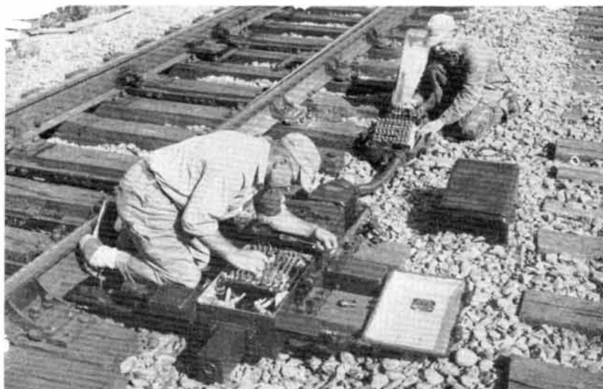
SWITCH MACHINE connections are checked at Gibson by William F. Gams, signalman (foreground) and Coit C. Seaman, signal helper.
