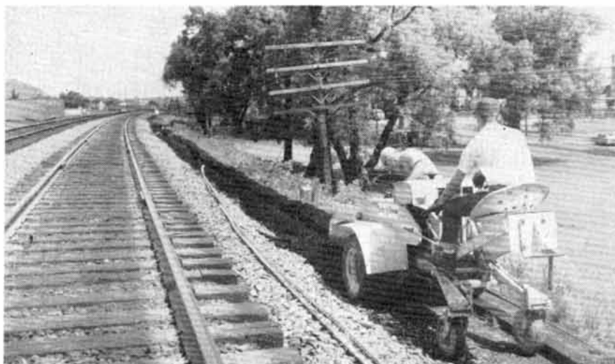
A DITCHING MACHINE is being used to bury cables wherever possible, saving untold hours of back-breaking labor.
