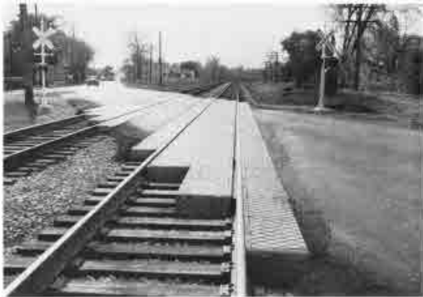
The new rubber crossing which was installed on Route No. 42 near West Salem, Ohio, where our tracks cross the highway is shown here as it looks after completion. The rubber crossing was featured in the November 1955 issue of the ERIE MAGAZINE.
