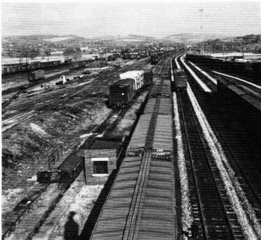
THE SCALE IN HORNEILL YARD , like all Erie equipment, is tested regularly. This picture shows a test weight car beside the scale house; to the right is part of Woodruff Yards, named for Robert E. Woodruff, retired chairman of the board.
