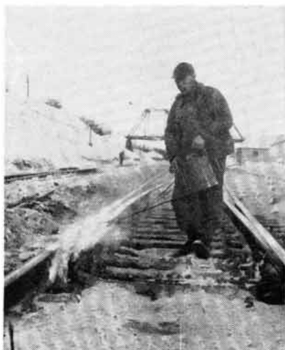
Assistant Section Foreman Salvatore Prisco thawing out a switch point with special snow oil burner. Switches are bottlenecks in a storm
