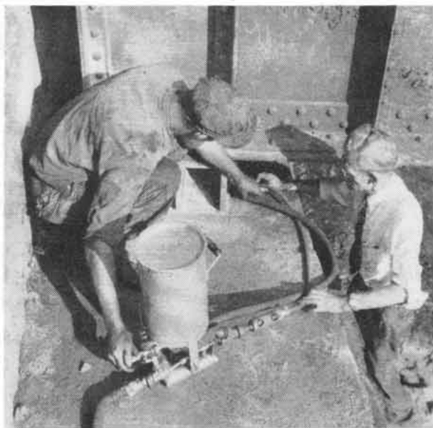
William Buchheister and Hans Johansen of the Dept. of Structures using a newly developed machine for forcing rust joint iron under bridge pedestals and bearing plates. Uneven bridge seats can be repaired without delay to railroad traffic by jacking and slow orders
