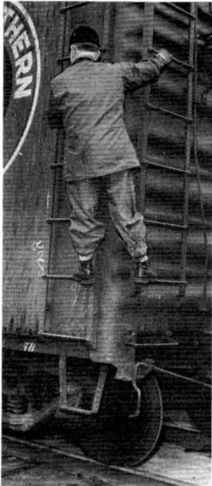
In climbing ladders, place feet slightly sideways with portion of balls of feet on the rungs. Demonstrating is H. G. Joyce, a yard conductor, while transferring from end to side ladder.
