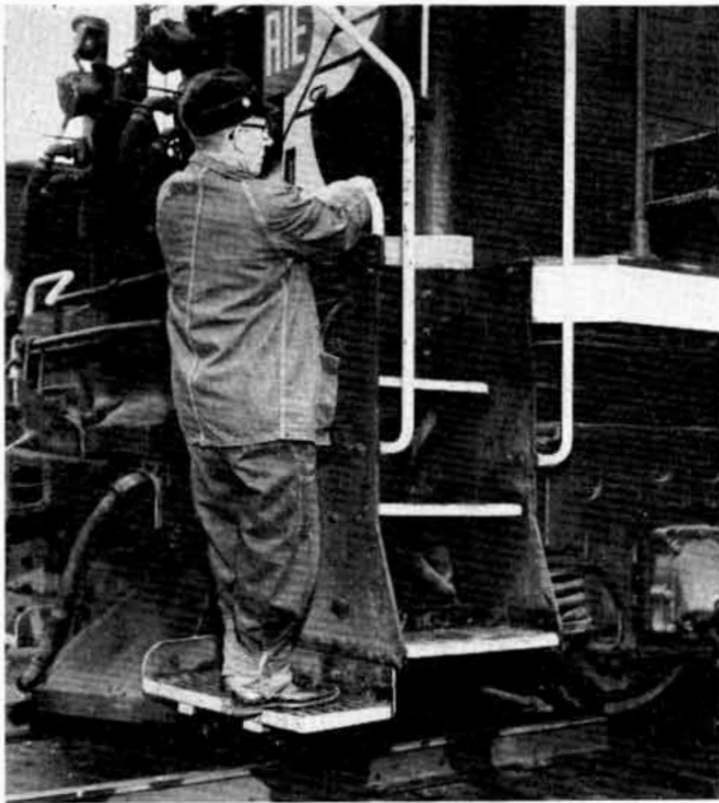
It is OK to ride the trailing foot-board of a moving engine like Yard Brakeman W. R. Phillips is doing here, but never ride the leading foot-board. If necessary to ride at the front of a moving engine, it is OK to ride the side step. Of course, you must always keep eyes open.
