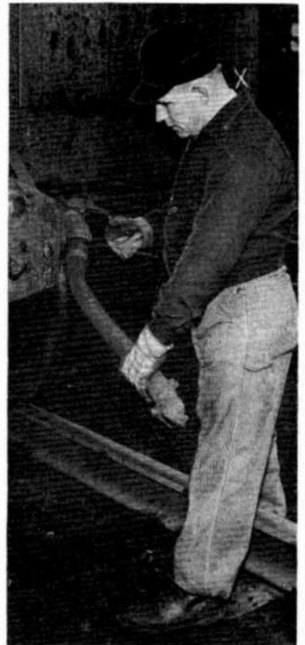
When opening angle cock, open valve slowly and hold the hose firmly so it does not lash. The demonstrator is V. M. Presco, yard conductor.
