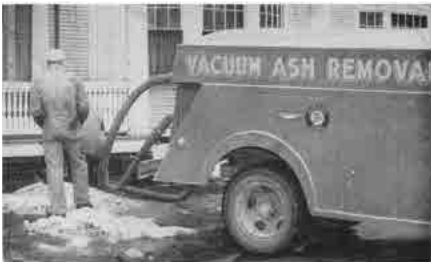
Above, a vacuum ash removal truck draws ashes from a furnace in a home which has a completely integrated automatic anthracite heating installation. With such a unit the coal is fed automatically, and the ashes are removed automatically. At right is a picture of an outside ash disposal unit for some automatic furnaces.
