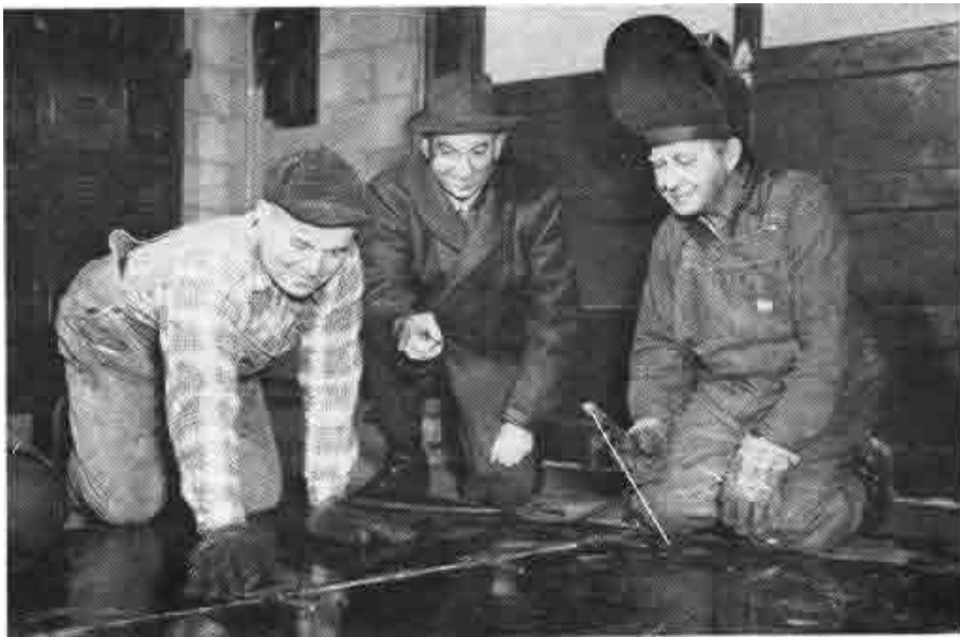
A DERRICK ENGINE ROOM DOOR is rebuilt at Hammond. Directing the job is John J. Urban (center), car foreman and wreckmaster. Carl E. Strykantz (left) air brake man, lays out hinges for Edward J. Furmanski, burner and welder.
