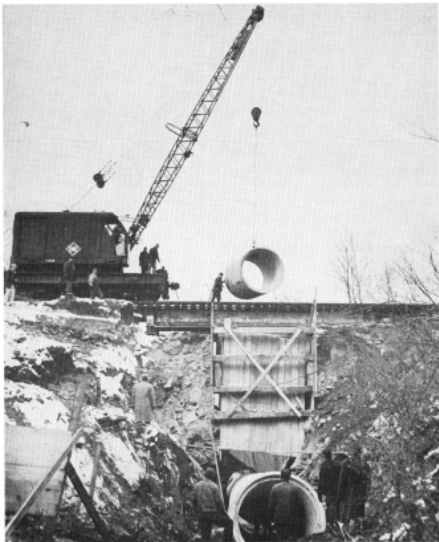
THE NEW CULVERT is of reinforced concrete pipe. Note the board lining of the shaft, here exposed, and the steel bridge span.
