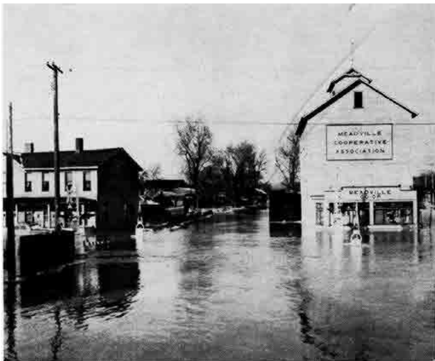
WATER, WATER EVERYWHERE, and very destructive when out of place. This is the main line through Meadville. The box car is on the Meadville Co-op siding, and the gates mark the position of Mercer Street. Note the water around the relay cabinets, a condition that hints of wide-spread hidden damage.
