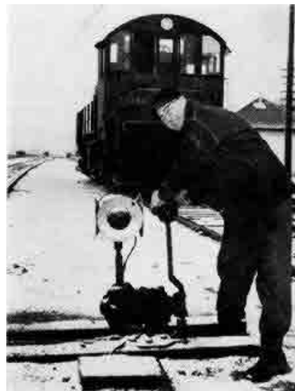
THROWING A SWITCH the safe way demands proper form. Here it is.
