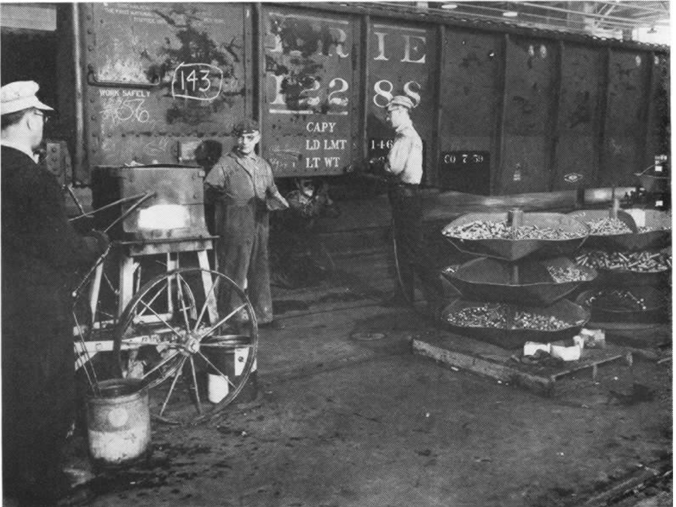
SIDE PANELS ARE RIVETED in place as part of the upgrading program.
