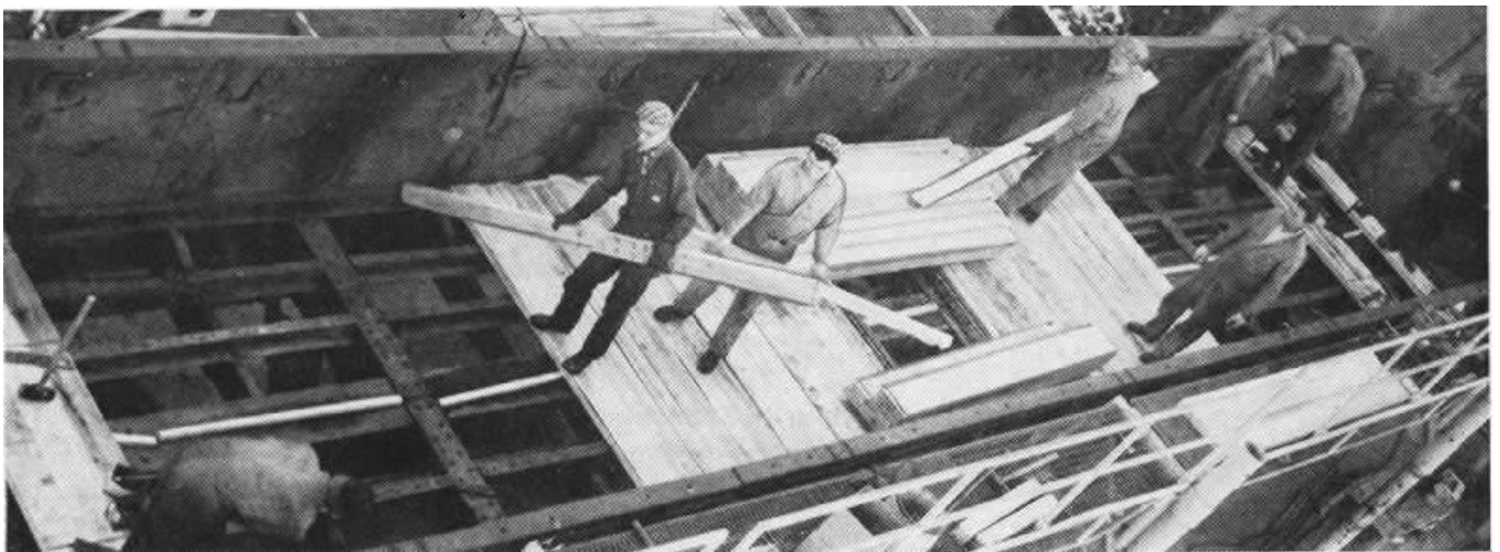
NEW OAK FLOORING IS INSTALLED in gondolas and jacked into place,
