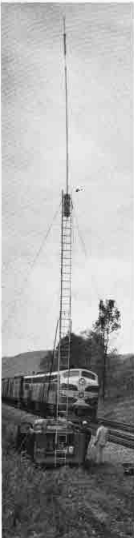
With temporary antenna erected, ground crew records train reception
