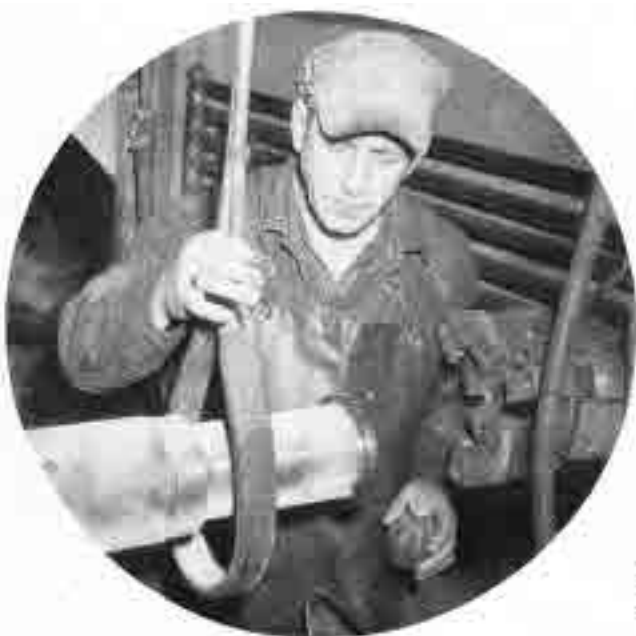
Paul Seaman, machinist, testing cur axles before they are fitted with wheels
