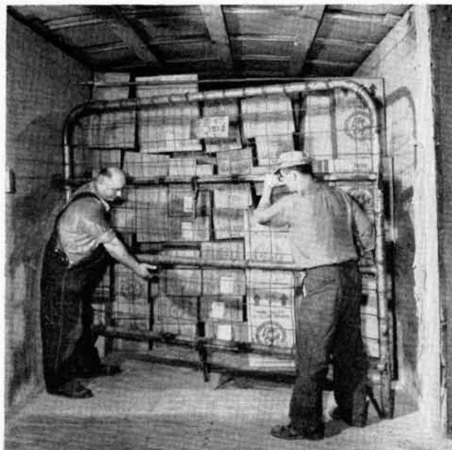
The Erie takes every possible precaution to avoid loss of and damage to LCL. Above are two pictures of the safety measures we have adopted. At left Eriemen install a steel bulkhead in a boxcar to prevent shifting of cartons in transit. At right, J. W. Fogarty, freight house
