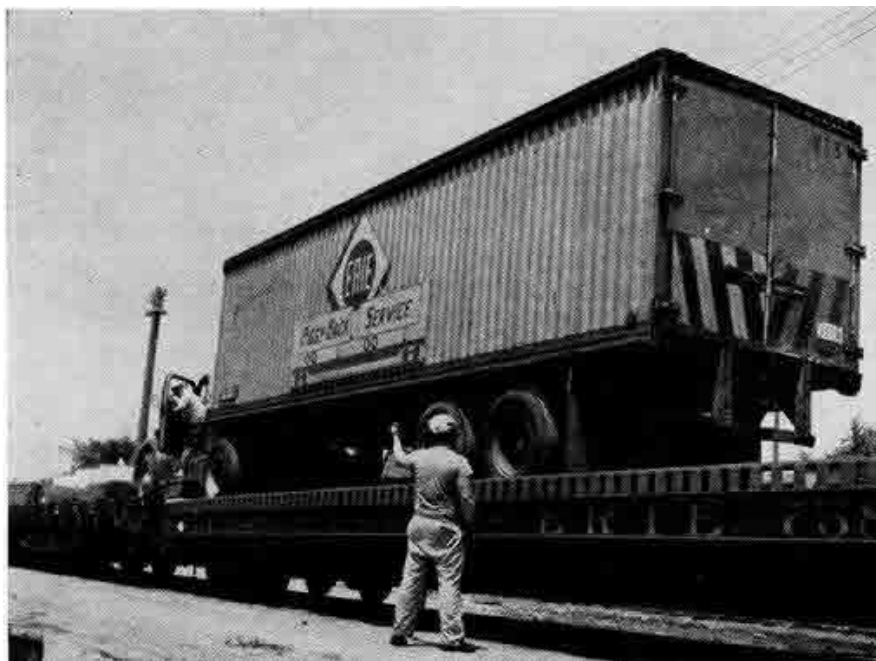
A TRAILER IS LOADED aboard a king-size Erie piggy-back flat built for this service.
