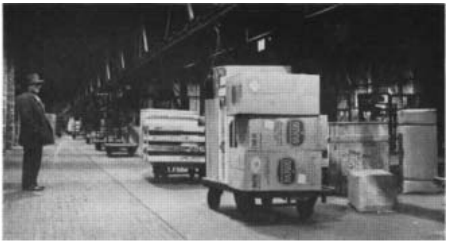
FIRST FLOOR TOWVEYOR LINE moves freight within the house swiftly, silently and efficiently.
