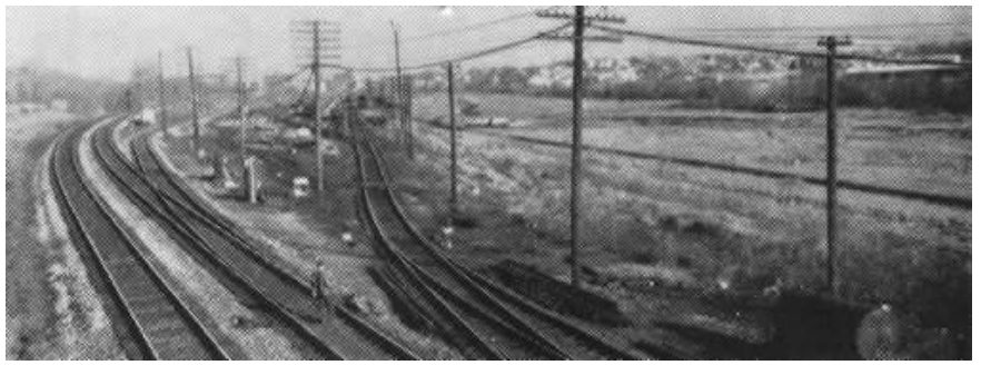
NEW JUNCTION POINT where Erie trains will reach the Boonton branch is marked by the No. 20 turnout where the man is standing; old yard lead to the right. The vast open space in the background is the site chosen by General Foods.
