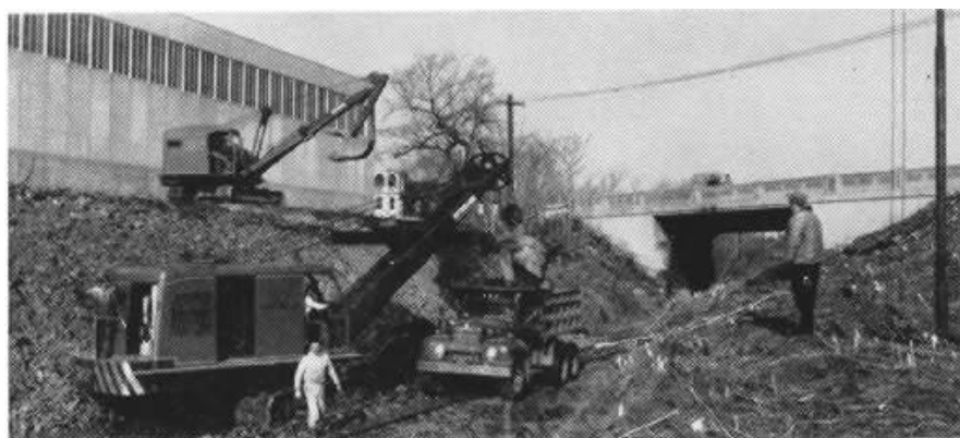
TWO SHOVELS WORK ON ROCK broken up by three-quarters of a ton of dynamite.
