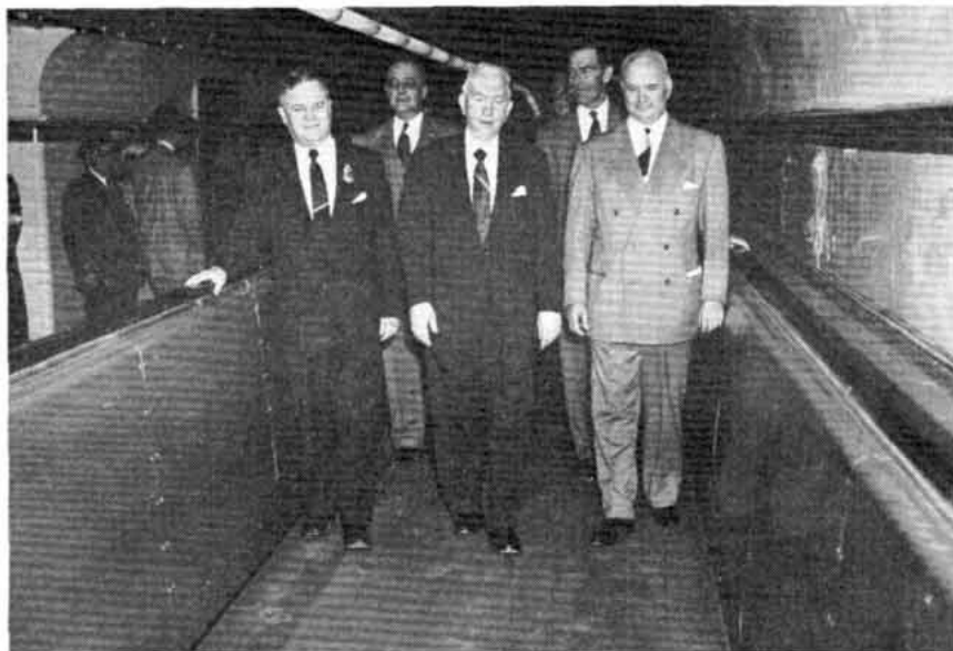
Officials take the first ride on the new speedwalk at our Jersey City Terminal. This is the endless rubber belt which carries commuters between our terminal and the Hudson & Manhattan Subway. This picture was taken during opening day ceremonies. In front row are, from the left, Bernard J. Berry, mayor of Jersey City; William Reid, president of the H. & M. and E. J. Thomas, president of the Goodyear Tire & Rubber Co. which was one of the co-builders of the new unique conveyor belt.
