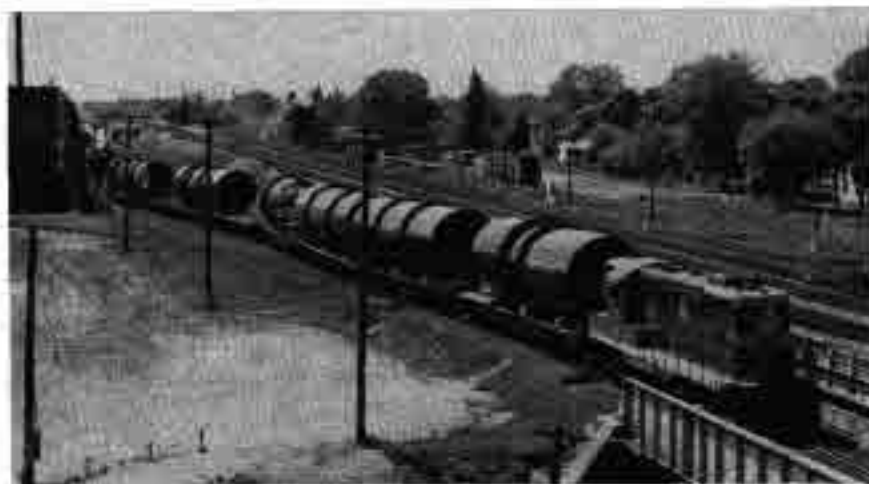
Bound for Fredonia, Kans., this string of 13 cars of rotary cylinder kilns manufactured by Alco Products, Znc., was handled by the Erie from the Alco plant at Dunkirk, N. Y. Most of the kilns were 16 feet 11 inches high from the rail and 13 feet two inches wide and required special handling.
