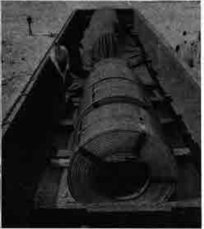
for 50 of our gondola cars. Note the cross-pieces for securing the steel coils in the cradle and the canvas.
