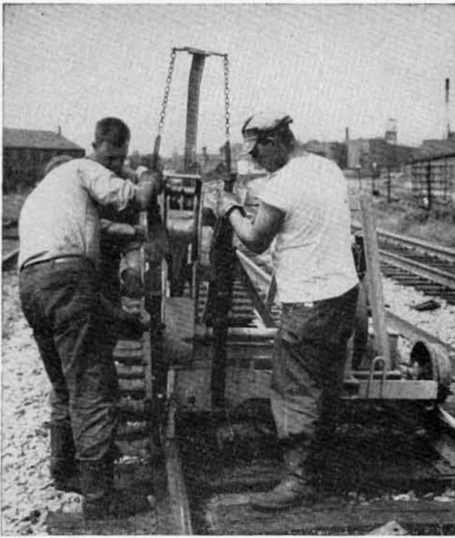
1. Using a mechanical spike puller, members of the crew which is installing the new rail remove the spikes from the old rail.
