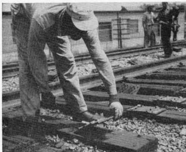
6. The tie plates are put in place next, then the rail is put in place by the locomotive crane (front cover).
