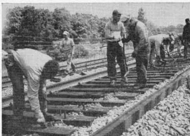
4. Wooden tie plugs are inserted into the holes left by removed spikes.
