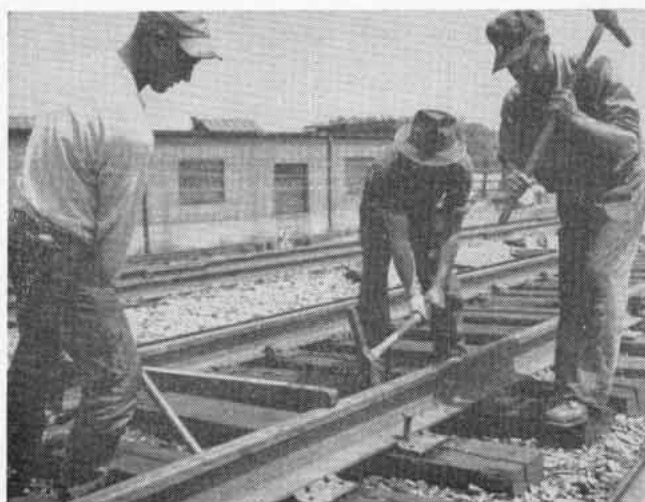
8. One spike on each side of the rail is driven manually every fourth tie and the rails are gaged for width again.
