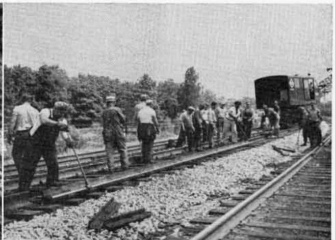
3. Two men with special tools roll out the old rail to make room for brand new rail.
