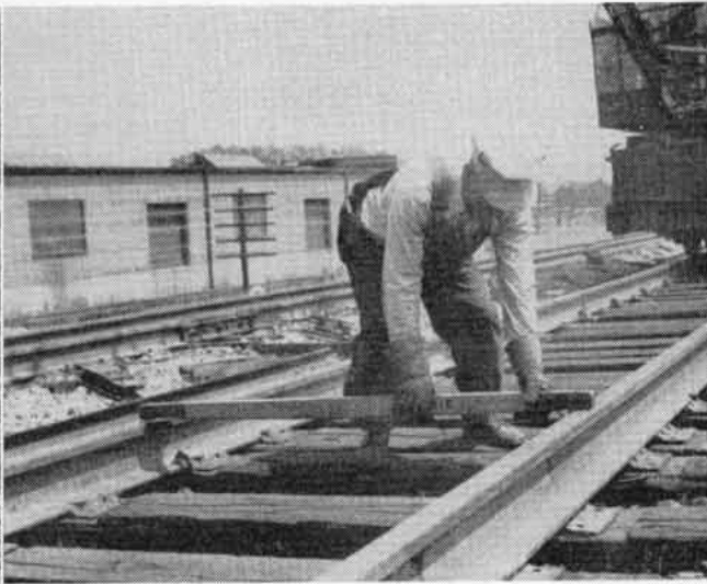
7. The new rail is gaged for exact width between rails to insure exact width.
