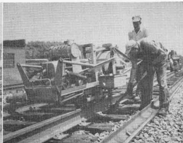
9. The mechanical spike driver comes along to drive the remainder of the spikes. The new rail now is ready for use.
