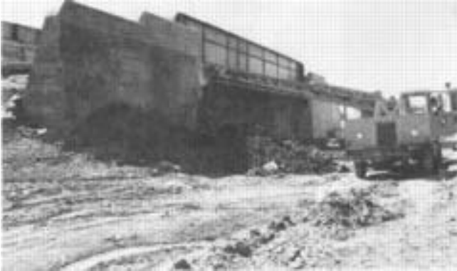
STRUCTURES ARE built, then the embankment is heaped up.
