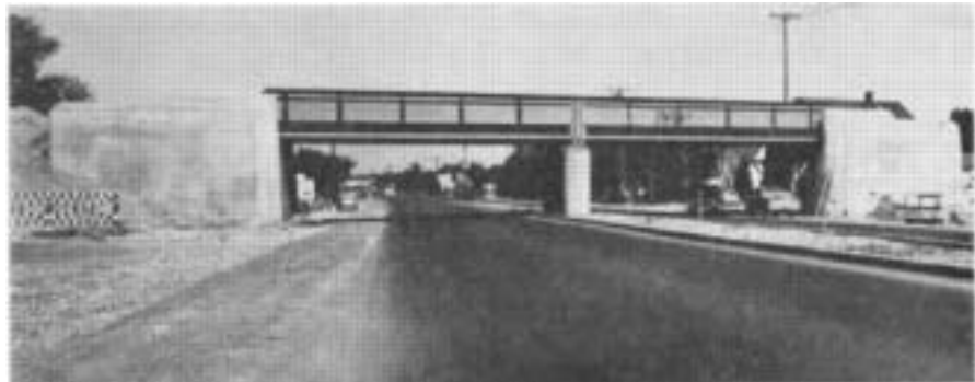
BUSY NIAGARA FALLS BOULEVARD rates a bridge of two spans.
