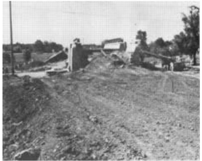
STRUCTURES ARE built, then the embankment is heaped up.
