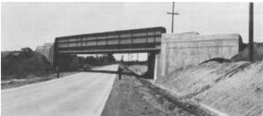
THIS IS THE BRIDGE OVER Walmore Road, one of several similar structures.
