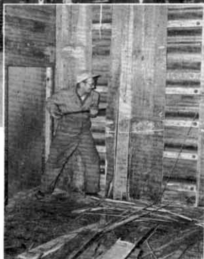
Old lining and flooring is ripped out to be replaced by new lumber.
