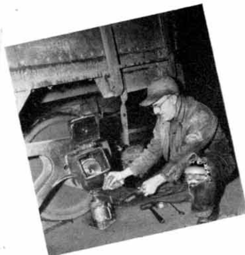
On the car renewal production line in the shop, the first step is to clean out and renew parts in the journal boxes.
