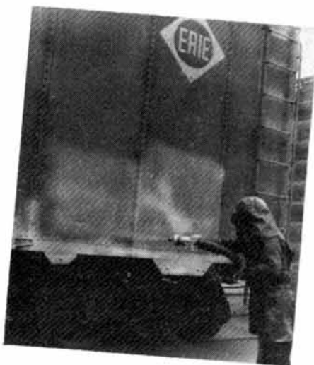
Sand-blasting of peeling paint preparatory to applying the new hot paint and stenciling.
