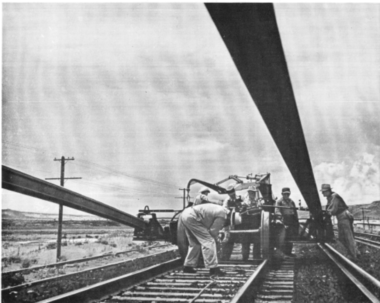
By welding sections of rail together in continuous lengths of steel, railroads often reduce track maintenance costs and give their customers a smoother ride. Above, workers lay the welded rail on ties.
