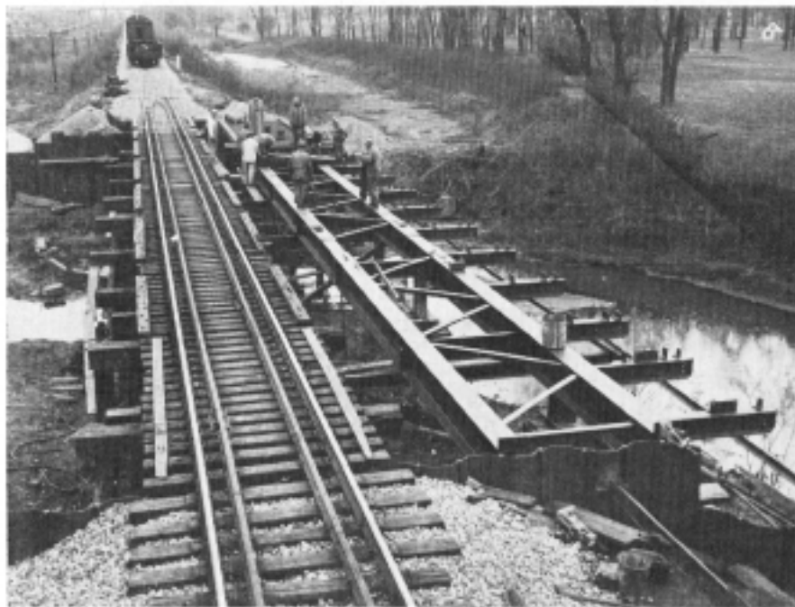
THE STEEL FOR THE DECK of the trestle lies on supports ready to receive the superstructure of ties and rails.
