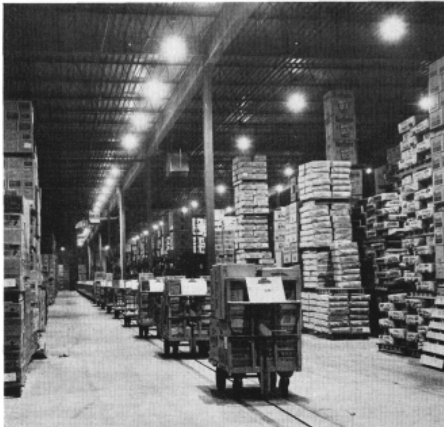
UNCANNY IS THE WORD for the way the stock trucks, loaded with orders for retailers, move silently and without human guidance from the storage area to the loading dock.
