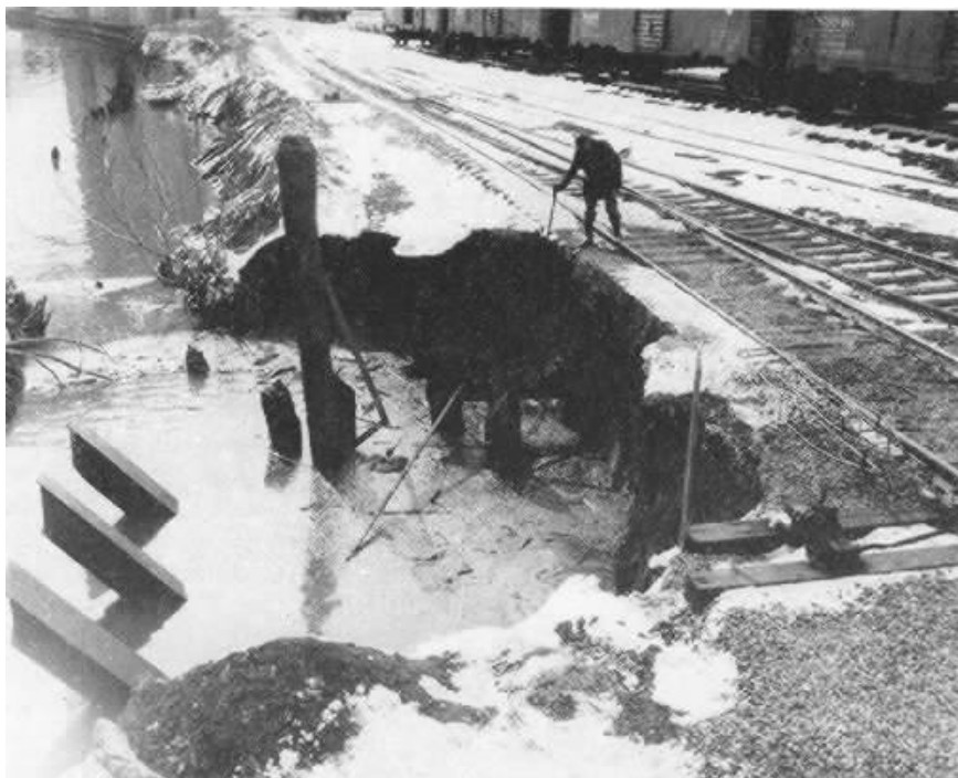
SOFT BANK OF THE CUYAHOGA , continually seeking to slip to the bottom of the river, collapsed some more as piles were driven into it.
