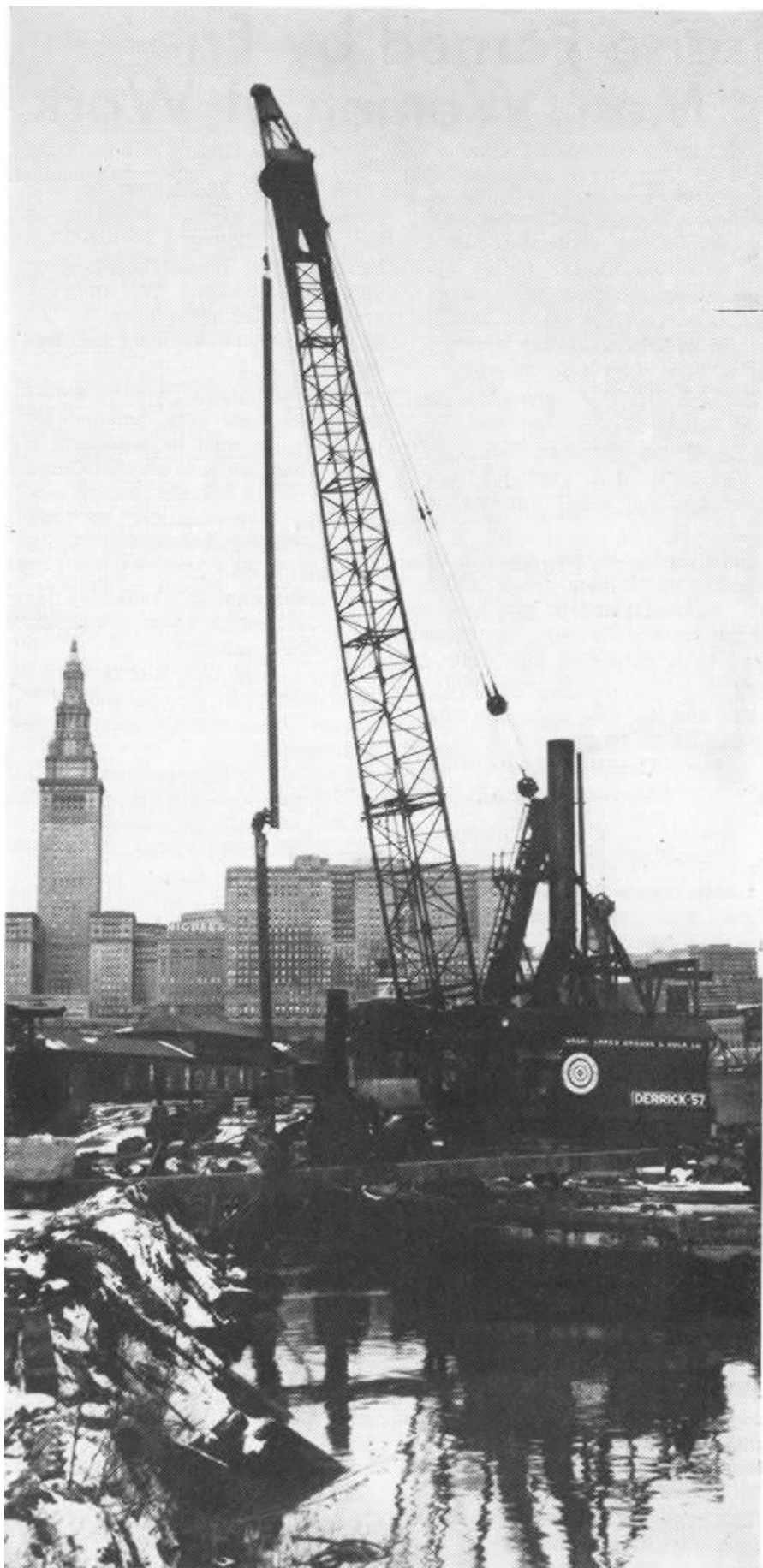
PERCHED HIGH ABOVE THE RIVER a workman interlocks two of the steel piles that will hold back the bank.
