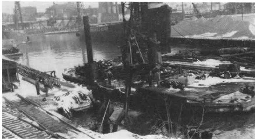
REMAINS OF ANCIENT TIMBER piling had to be removed before the new sheet steel piles could be driven.
