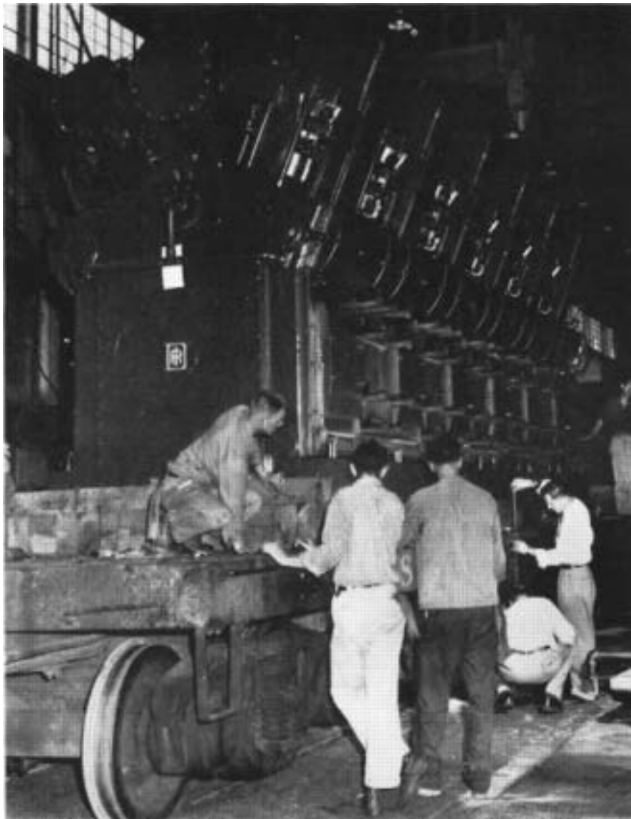
FIRST OF ITS SIZE , this huge compressor was built by Ingersoll-Rand Co. at Painted Post and shipped to a gas pipe line company via Erie. The shipping weight of the machine was 210,000 pounds.
