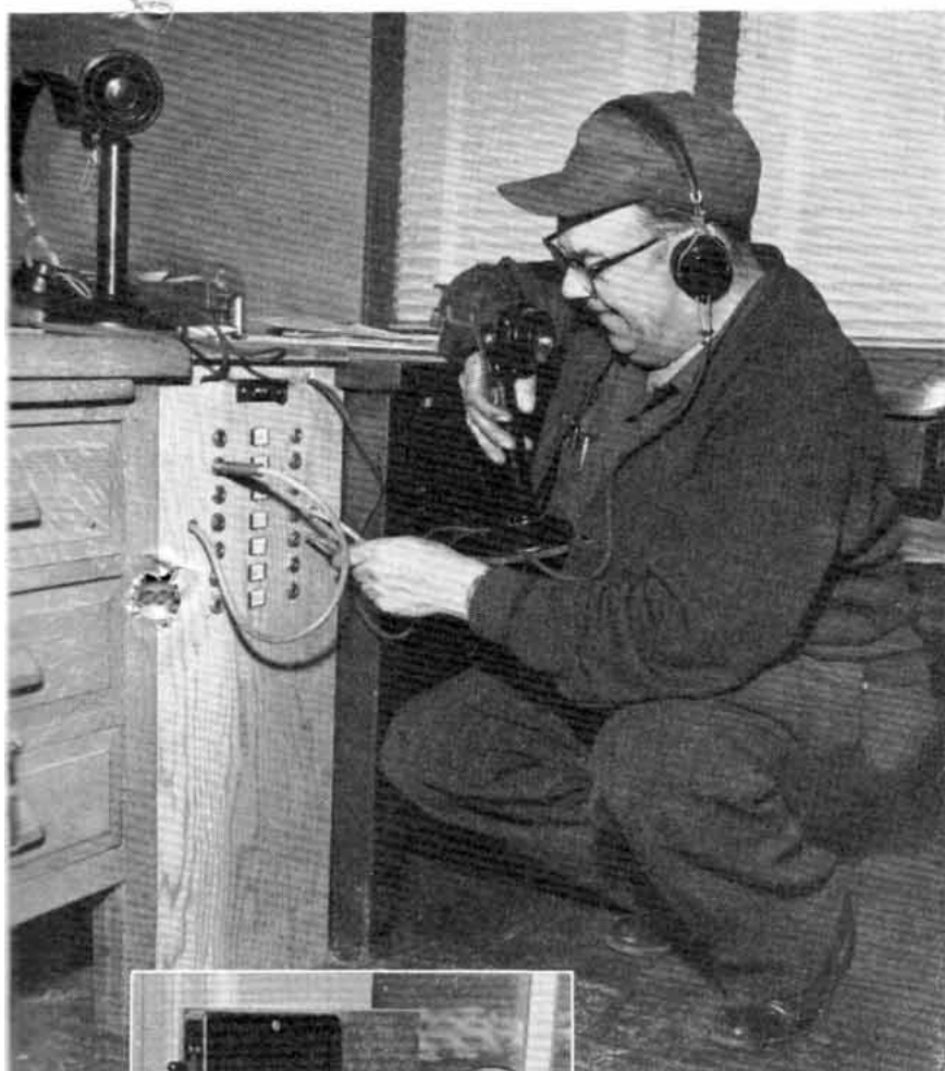
At left, Hubert Kelly, division telephone supervisor, checks one of the new jack boxes he has installed in the Huntington offices. New lines can be added easily to this type box. Inset is the old type box which has a limited area for new lines.
