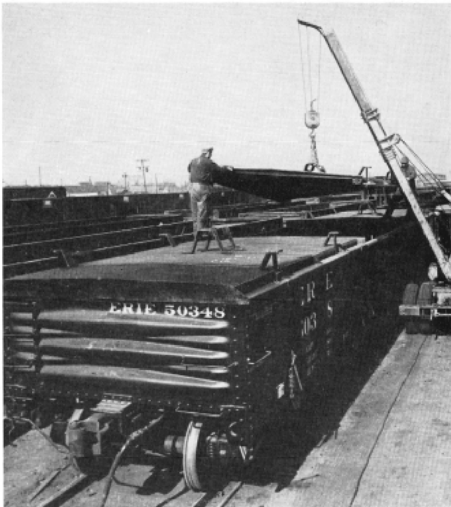
THE CENTER SECTION GOES ON LAST , and seals the car against the weather. Note the piling brackets welded to the sections.
