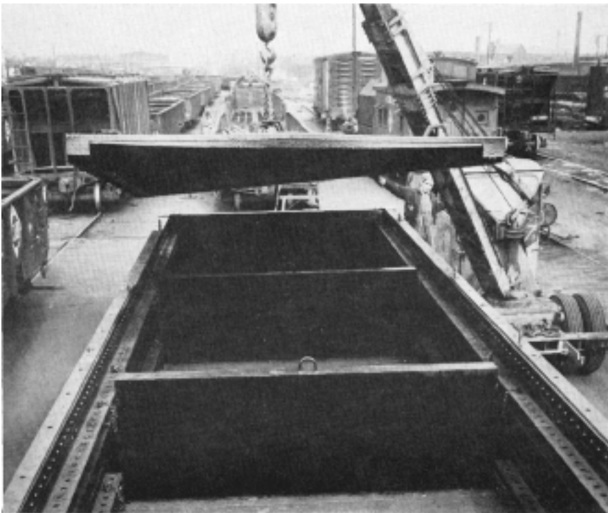
END ROOF SECTIONS ARE LOWERED into place before the center section.
