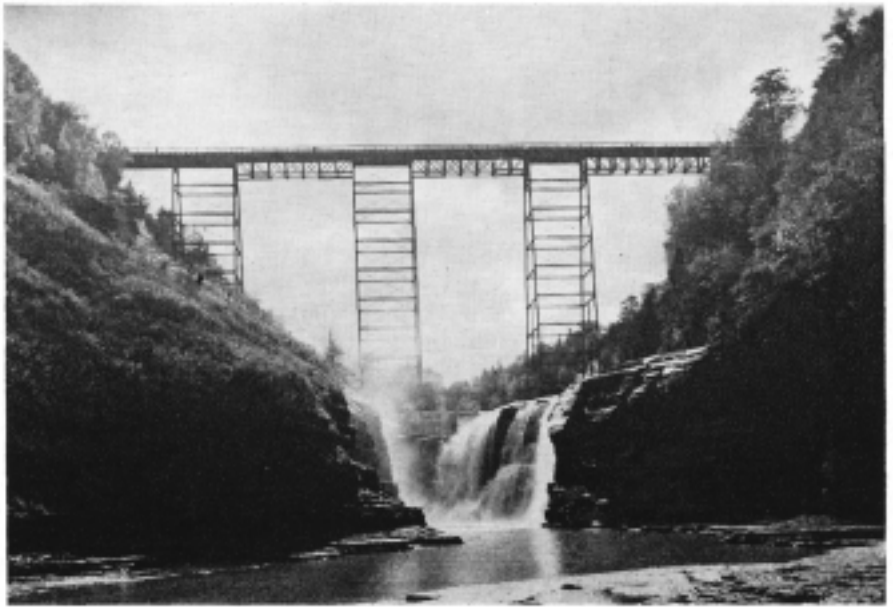
AT THE FALLS OF THE GENESEE the Erie crosses river and gorge on a viaduct more than 200 feet above the river and more than 800 feet long.
