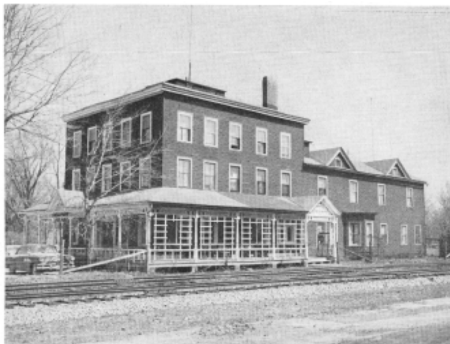
THE OLD STAGE HOUSE at Attica spans two eras. The coaching inn was remodeled for railroad use by the addition of a side porch and the railroad office wing (with bay window) at the rear of the old hotel.
