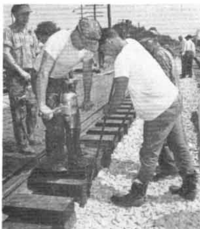
Workmen install wood risers over ties for the rubber crossing. The rubber slabs, a little more than three inches thick, then rest on these risers.
