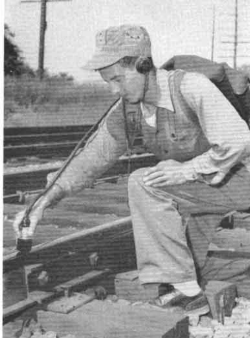
Anthony J. Ceja, signalman from Warren, Ohio, demonstrates use of the Audigage flaw detector at a joint bar.
