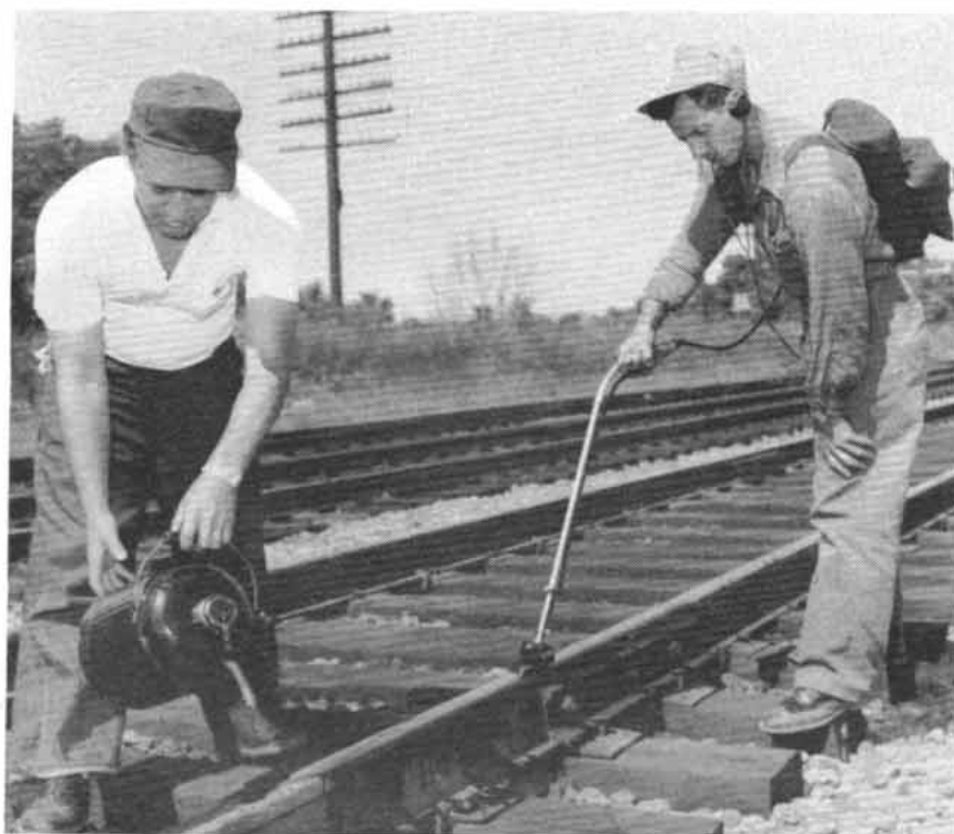
While Joe Byrdy, signal helper, applies a film of oil to the rail to improve efficiency of the instrument, Anthony J. Ceja, signalman, demonstrates use of the Sonirail flaw detector.
