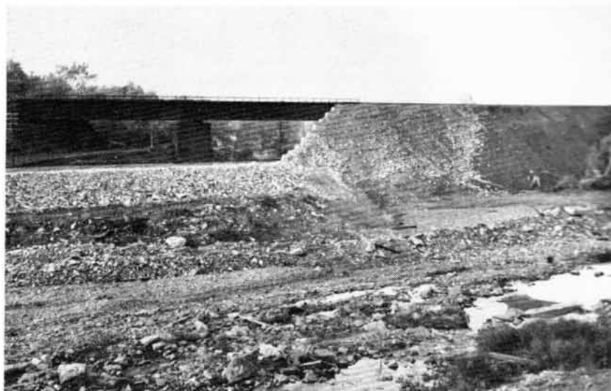
THOUSANDS OF TONS of new fill went into this embankment to replace one lost during the floods that hurricane Diane dumped on the Wyoming division.
