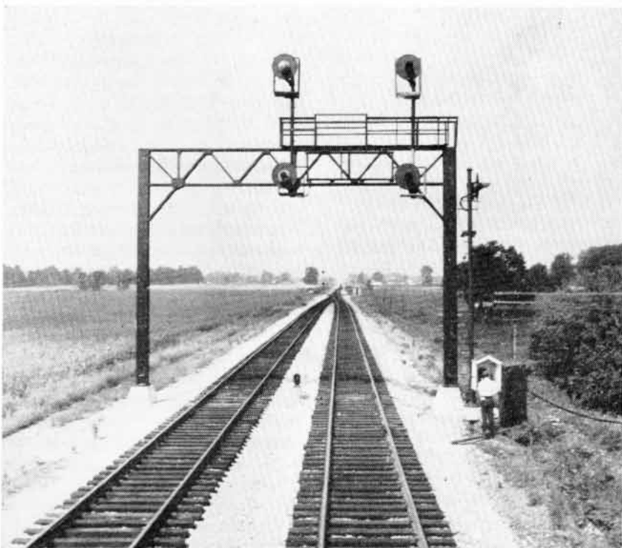
NEW SIGNAL BRIDGE AT MP 148.20, near Disko is sign of modern railroad practice.
