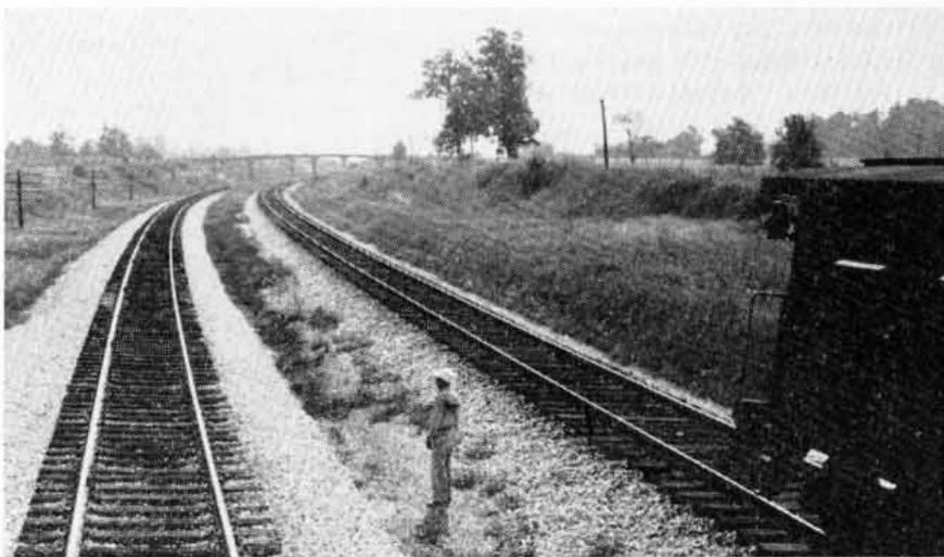
GRADE SEPARATIONS were part of the modernization program of 1911-1916. Today they enable freight trains to run at speeds undreamed of then. Here the two tracks are about to reach the same level, just around the curve and under the highway bridge.
