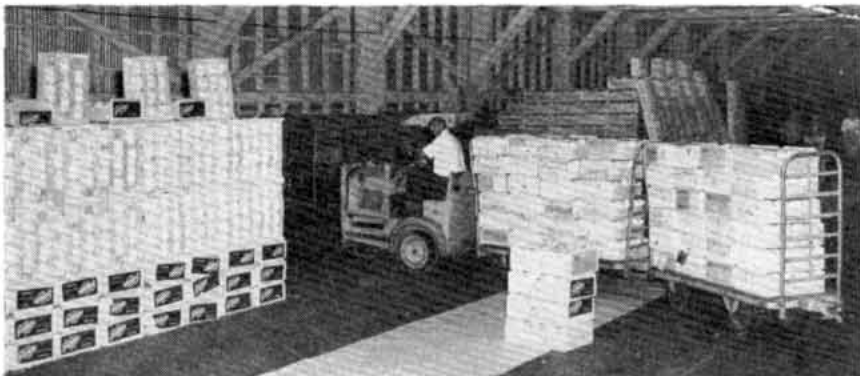
One of the tractors brings two trailer-loads of fruit into a display area. The tractor immediately picks up two empty trailers and takes them back to a refrigerator car to be loaded.
