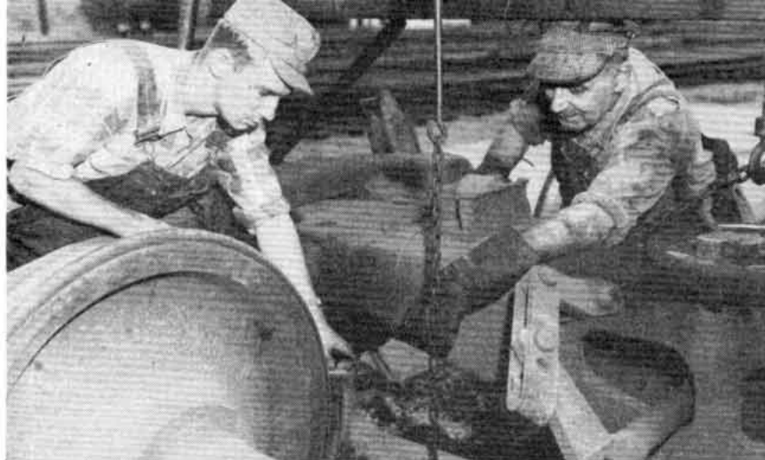
On one of the repair tracks, Dave Evans, car repairer helper, and Joe Jaworski, car repairer, were busy replacing a set of wheels on a truck.
