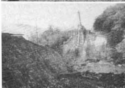
Above is a view of the new timber and steel trestle bridge at Parker's Glen, Pa., where the biggest washout occurred. Inset is how the same scene looked just a few days after the flood.
