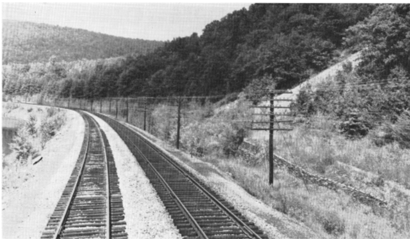
FREQUENT LANDSLIDES forced the Erie to relocate the river at Boucheaux in order to move its own right of way. The stone revetment of the old embankment may be seen at the right of the picture.
