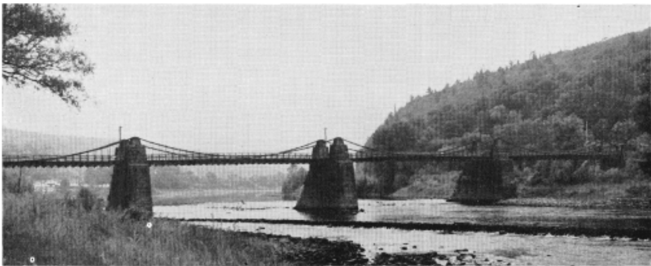
THESE MASSIVE PIERS once carried the Delaware & Hudson Canal across the Delaware at Lackawaxen. Today they support a highway bridge.
