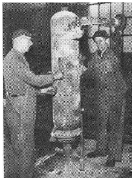
PREPARING SEPARATOR for pressure tests are Floyd Martin , machinist, and Edward T. Sullivan , pipefitter.
