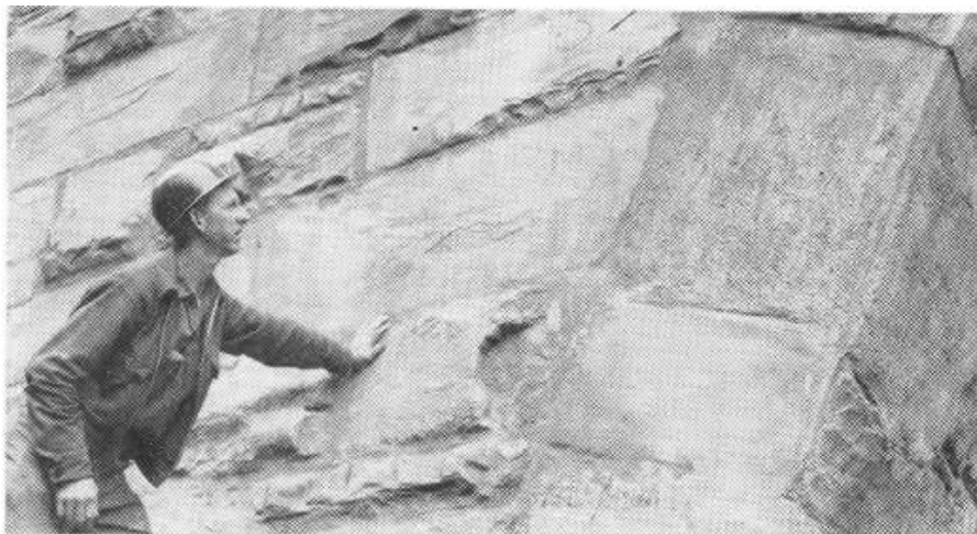
CLEANED AND REPAIRED, the masonry is subjected to an inspection. The repairs are expected to last at least a century.
