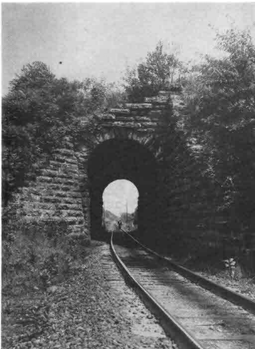
DAYTON TUNNEL, PERHAPS THE SHORTEST on the Erie, has a barrel vault only 90 feet long. The B&SW runs through it on high quality trackwork; the Dunkirk Branch passes over it. The stonework, still solid, strong and sightly, is a tribute to the workmanship of the masons who built it.
