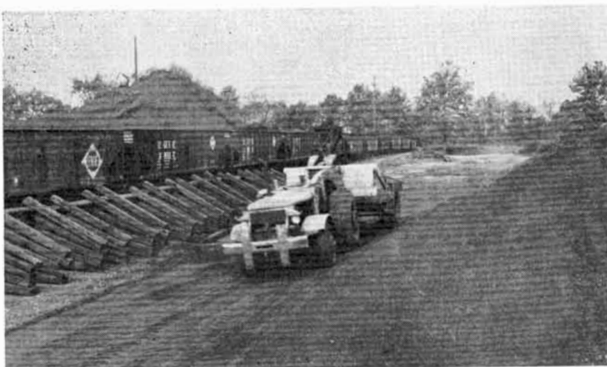
ENROUTE FROM STORAGE to dumping area, a scraper passes between the rapidly forming pile and the cribbing that marks its eventual limits.
