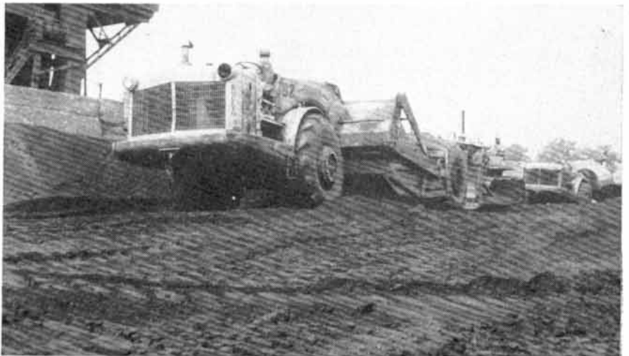
THE PILE SINKS QUICKLY as scrapers and bulldozers move through it.
