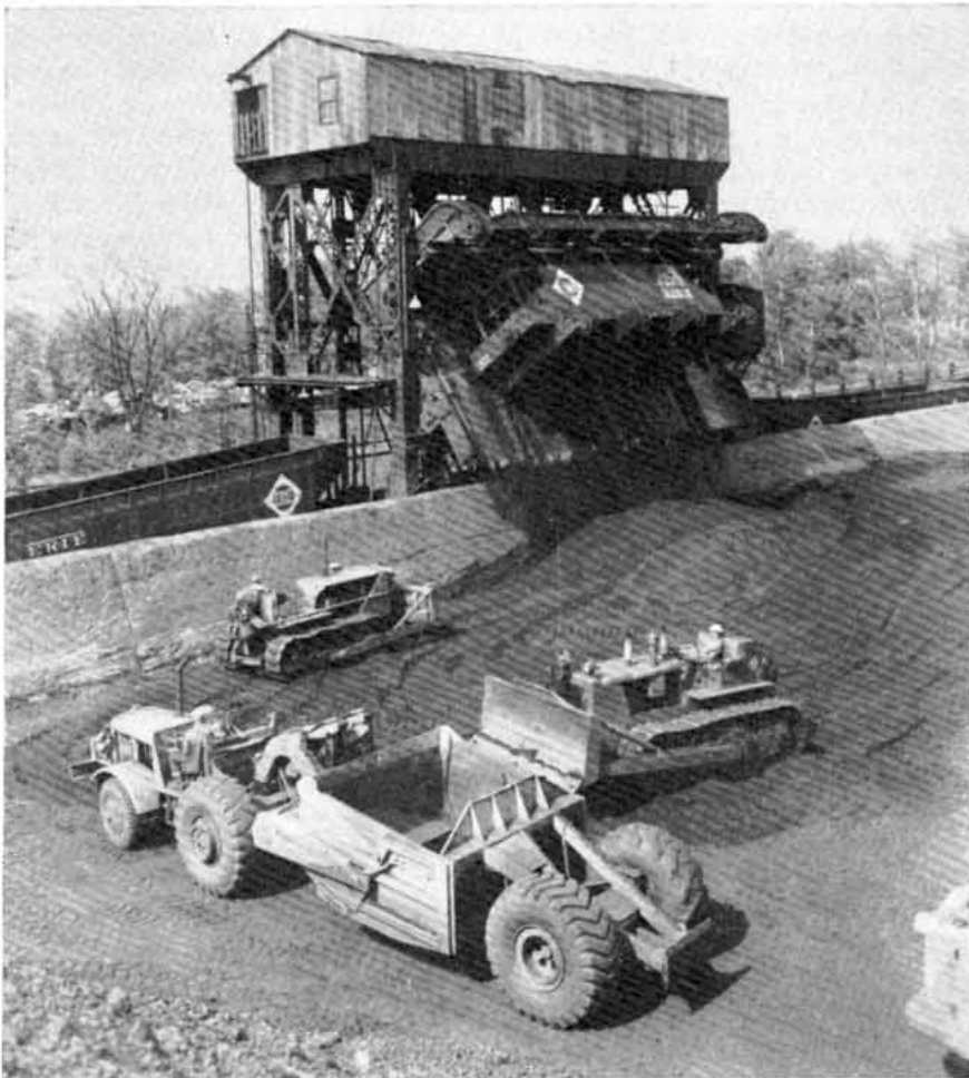
A BULLDOZER DRIVER stands by, ready to move in and smooth a path over the pile as soon as the last of the ore falls from the car.
