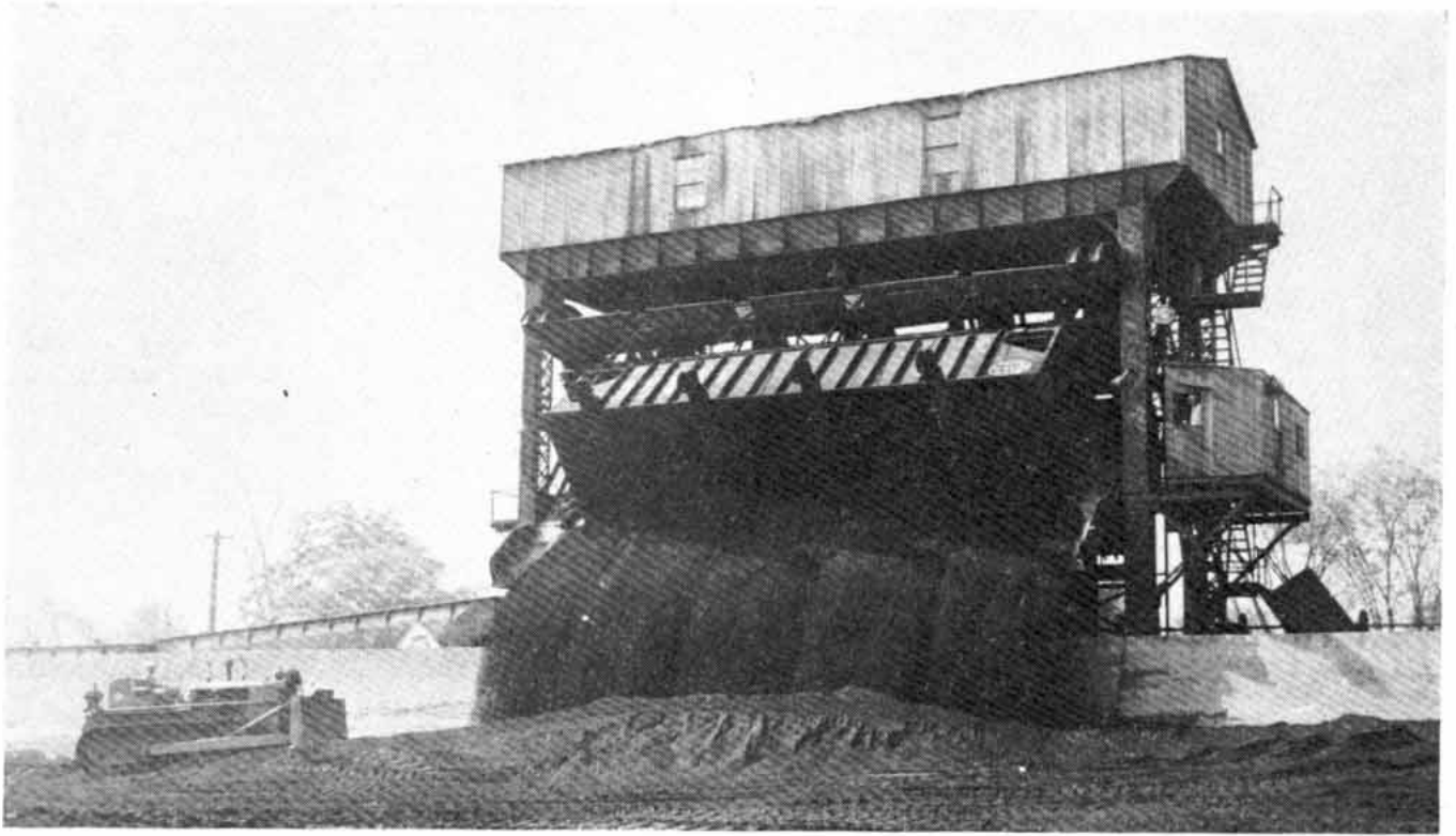
SEVENTY TONS OF ORE pour from the car as the dumper tips it over.
