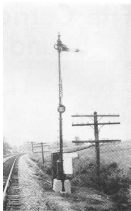
NO DOUBT is left of what the detector found by this signal. Note the telephone box beside the line, from which the crew may call the dispatcher.
