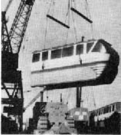
Each monorail train is made up of 4 cars like this one being moved from lighter to flat car in E-L Hoboken yards. Cars average 13 tons each.
