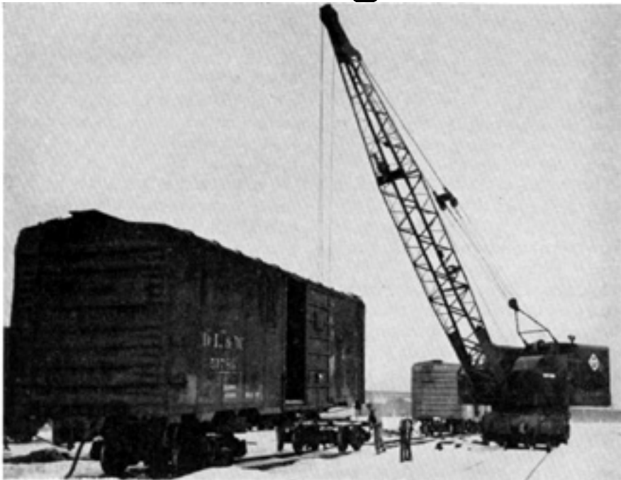
FIRST STEP in the rejuvenation process for a box car is the lifting of the car body from the trucks. Then the trucks are moved toward the center of the car, and the body lowered for the trip through the line.
