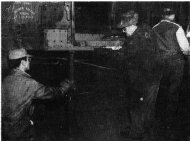
4 Here the punched and shaped reinforcing plate is applied to the car in a "fitting-up" position. Operation is being performed by E. F. Deramo, Jr. (L) and P. J. Romaniello, while to the right, J. A. Hoizan goes into action with a torch.
