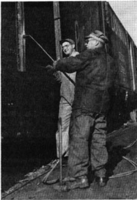
1 One of the first operations takes place outside the shop, in the strip yard, where parts of the cars can be straightened after being heated by a flame-throwing torch. Here H. E. Nichols (L) and P. J. Glasso are working on a box-car door frame.
