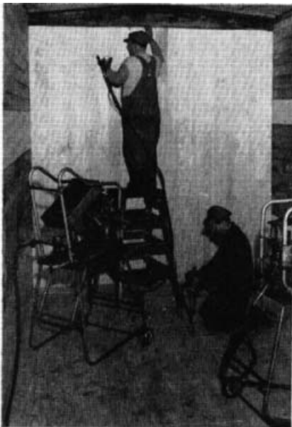
8 Meanwhile, back in the boxcar, D. A. Petruolo (L) and R. A. Stallsmith are refurbishing the interior side and end walls of a car. Walls do not suffer as much hard use as floors do, and so a patch job is done, rather than an entire relining. Light-colored areas in picture are new lumber.
