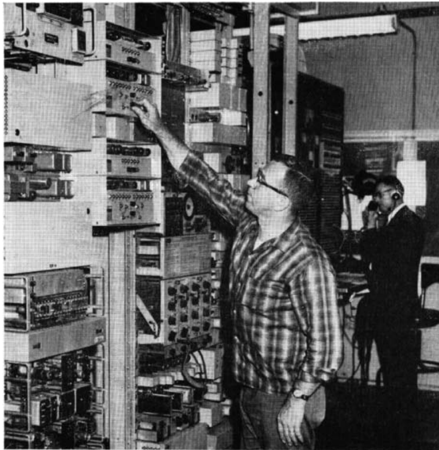
"Brains" of Erie-Lackawanna's new Communication Center at Hoboken are these electronic devices. In foreground is D. C. Gregory, lead constructionman, who handled a good deal of the installation. At rear is E. D. Dempsey, assistant supervisor, communications, at the test board. Each of the various bays handle the carrier system voice and telegraph channels.
