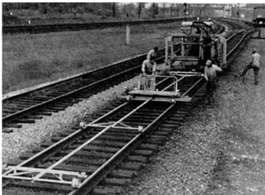
TIGHT LENGTHS OF PIANO STRINGS stretch above the rails to indicate low spots in the track. In this long view, foreman Joe Minelasco and trackman Joe Perko move the surfacer along the tracks, while Edward Innes , left, and Chester Marks use forks to place ballast around marked ties. Ballast tamper operated by Lester Quails follows up to complete the job.
