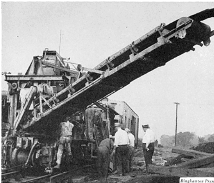
ABOVE: Hungry jaws of 'bailas-ter' chew away at roadbed beneath ties and track. Note depth of cut.
