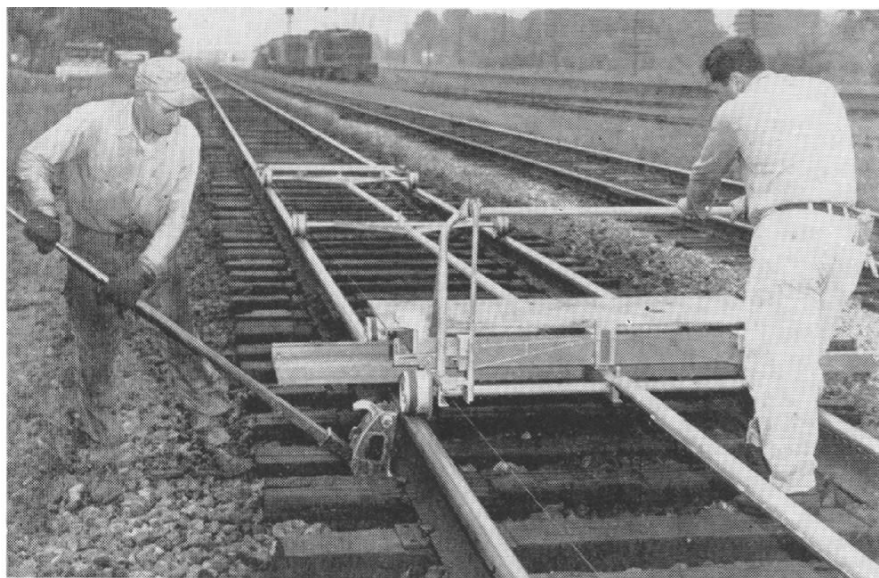
JOE MINELASCO , track foreman, right, checks the indicator dial on the track surfacer to determine if track is level, while Joe Perko , trackman, awaits instructions. Machine can measure dips as small as one-eighth inch.
