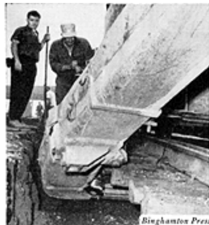
ABOVE: Hungry jaws of 'bailas-ter' chew away at roadbed beneath ties and track. Note depth of cut.
