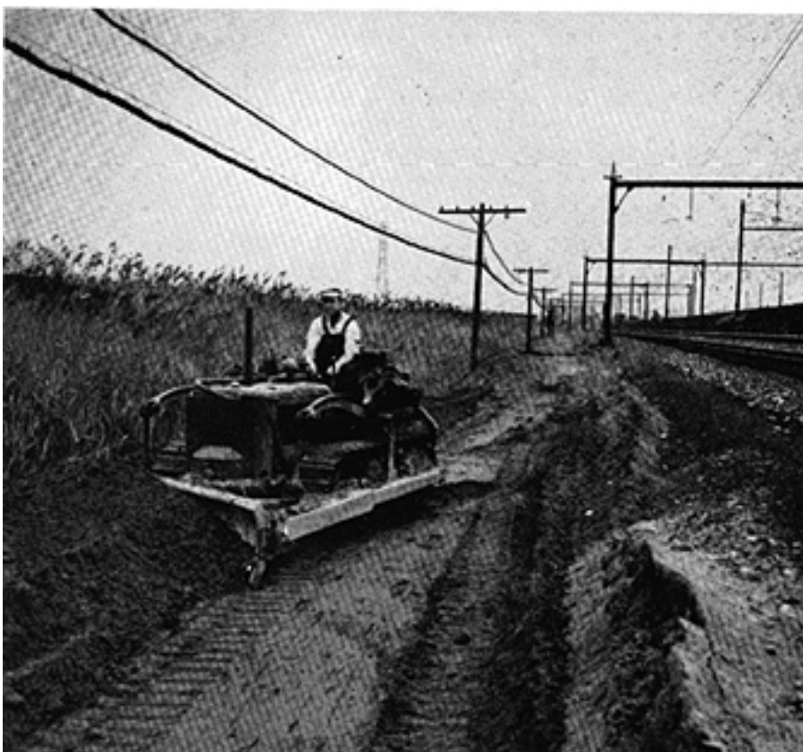
After material was unloaded bull dozer leveled off the road. It is 25 feet wide and elevated two to three feet above the ground level.
