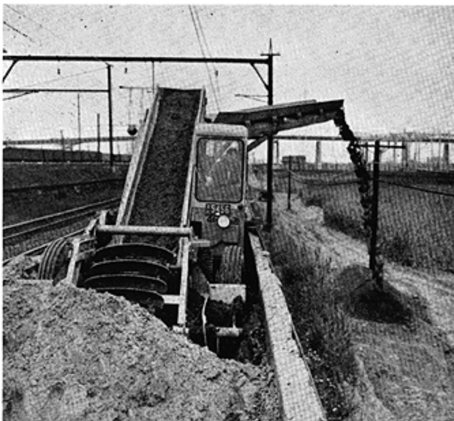
Self-propelled vehicle moved through gondolas to unload material for road across the meadows. This material came from Secaucus yard where construction work was in progress.
