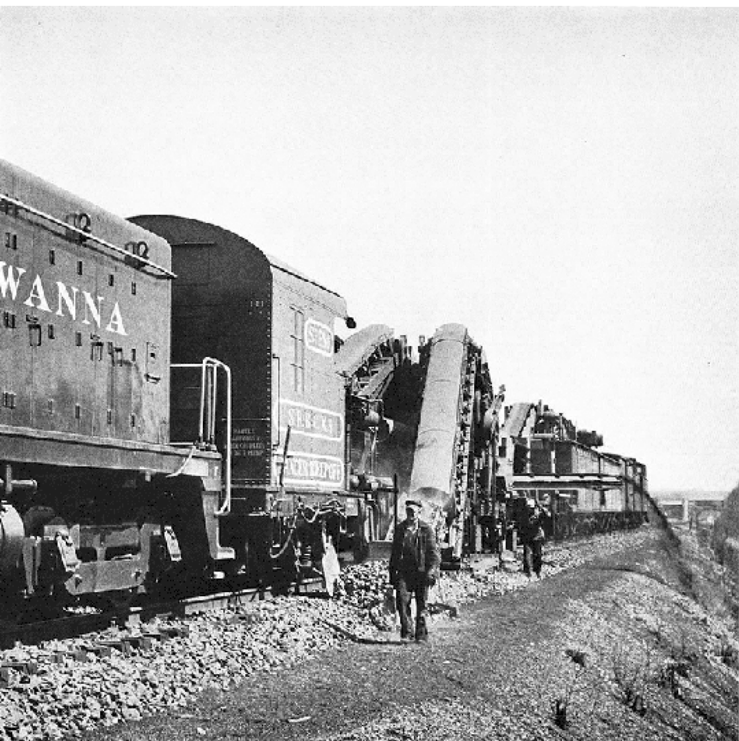
Working on the Lackawanna last month, and continuing at various times and places this summer, is this big ballast cleaning car. The machine scoops up the ballast, shakes out the dirt and throws it out to the side, replaces the ballast neat as a pin.
