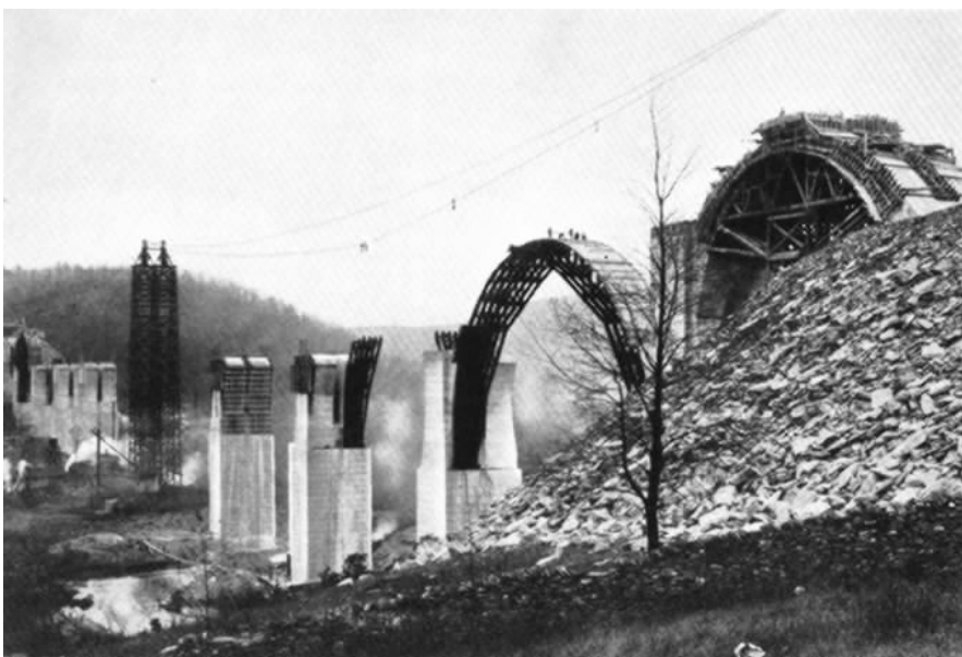
Here is one of the sectional side forms for the blocks of the 180 foot arch. After concrete was poured and had set, form was moved over to other side of pier. Abutment arch at right was entirely buried by approach fill.
