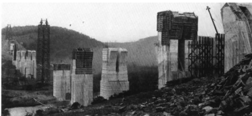
Piers here are ready for the arch rings. I-beam grillage was fastened to the piers by anchor bolts set in the concrete.
