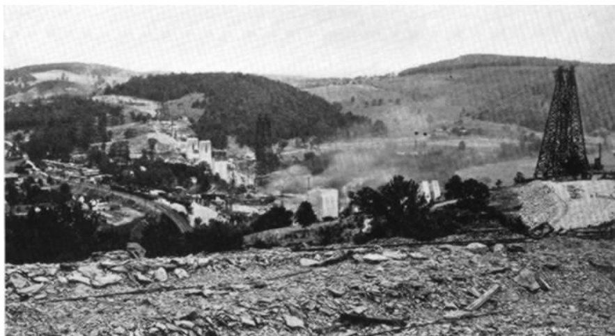
The tall wooden towers which can be seen here supported the cables which carried the materials for the construction of the viaduct.
